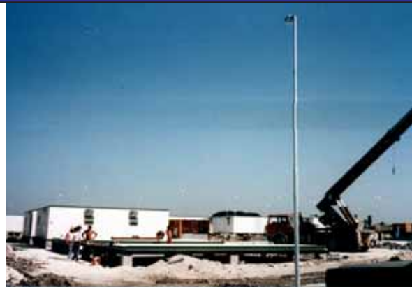
Porta-cabin Construction - May 1983
