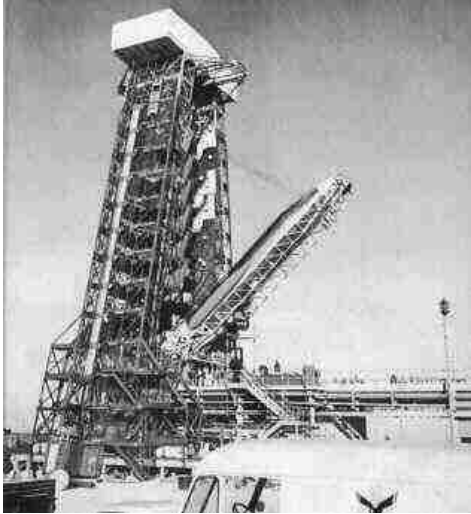
Atlas Installation in the Gantry
