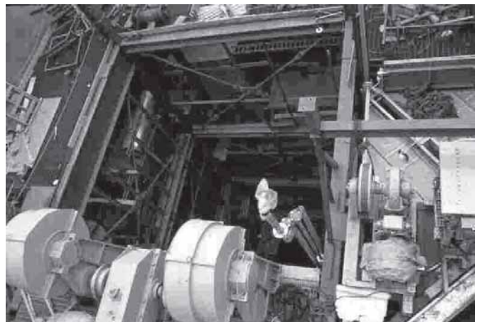
Atlas F Silo - looking down
