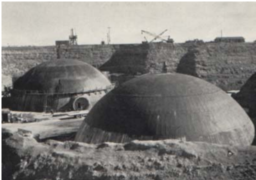
Power house and control center domes
