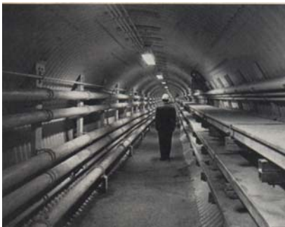
Tunnel to missile silos
