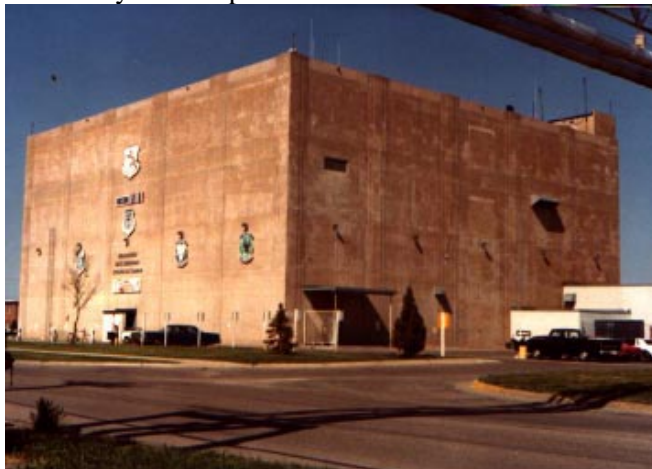
Building 306, the home of the 321SMW/MG at Grand Forks is gone - several members sent information about its demolition. Many of us spent many hours in this old blockhouse.
