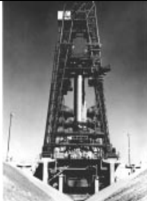
Atlas in Gantry at Vandenberg in the early days
